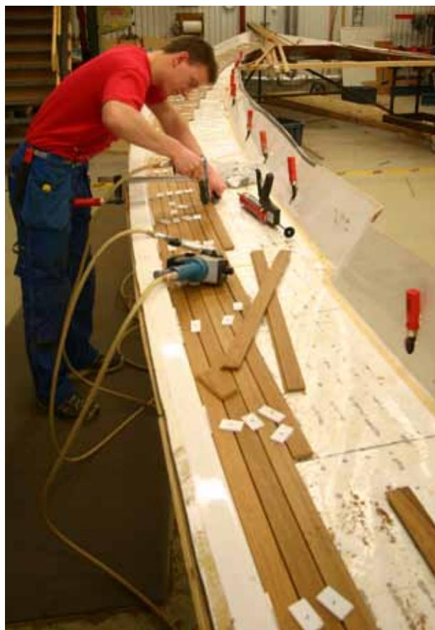
*Teak deck, handcrafted on a template outside the boat, 10 mm thick solid wood, from 34 ft vacuum glued without screws to the GRP deck*
